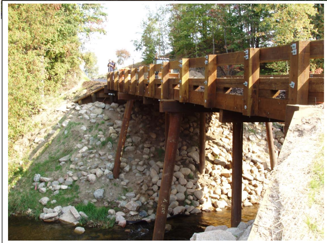
The completed structure includes paved approaches, runoff controls, and a clear span of the stream channel with virtually unlimited space for stream flow beneath the structure.
