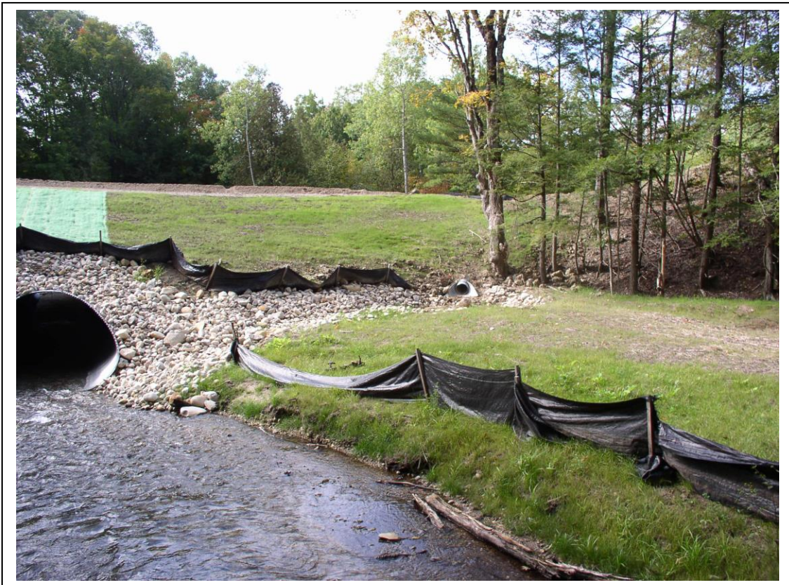
Small, short culverts caused both a plunge pool at the outlet and embankment erosion along the road shoulder.
