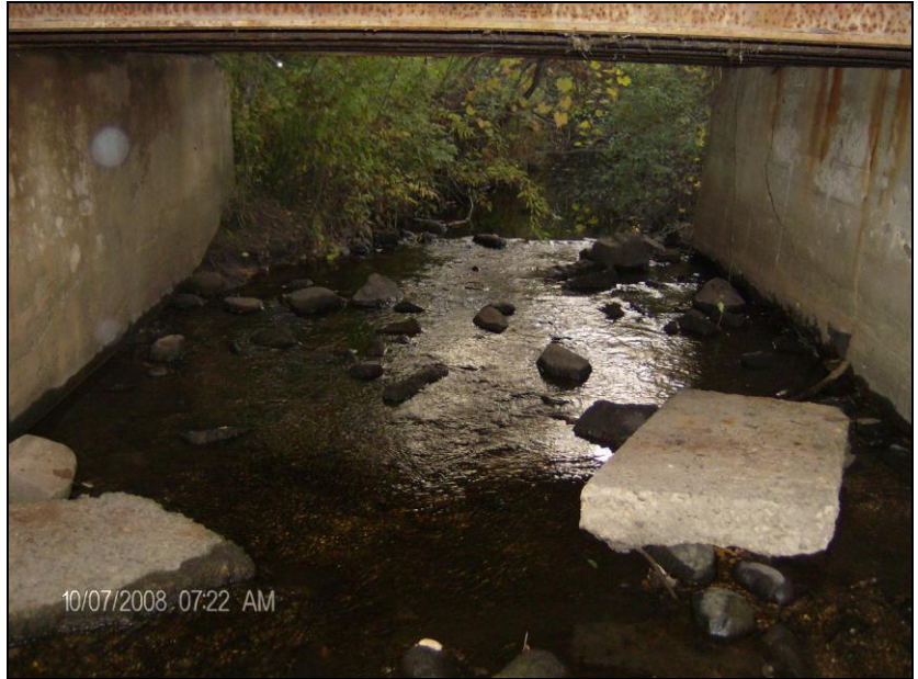
Bridge deck – after
