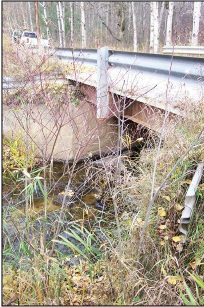
Bridge deck – before
