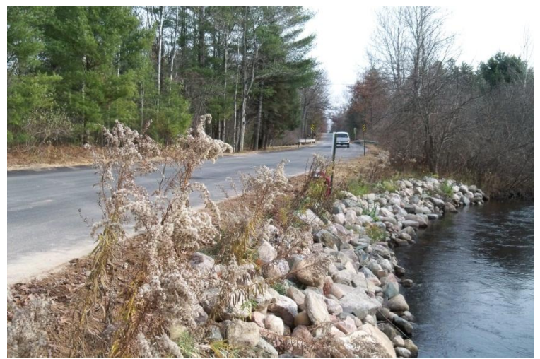
Fieldstone placement now stabilizes the streambank
