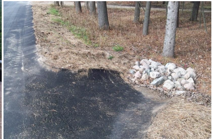
Sand from the road constantly washed into the river; 8 spillways now help direct runoff into uplands.
