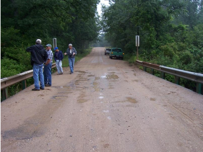
Sand from the road constantly washed into the river; 8 spillways now help direct runoff into uplands.
