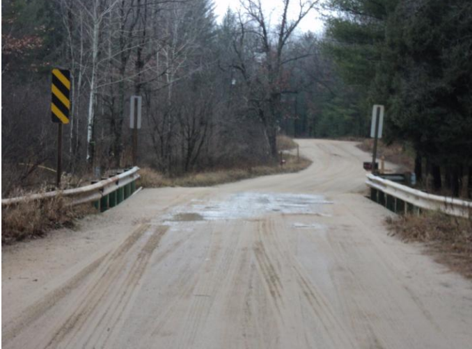
Rain & snowmelt on sloped approaches pooled at bridge. Now pavement & curbing limit & control runoff.
