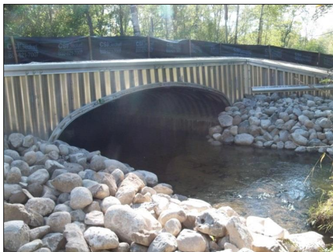
Culvert and rock work
