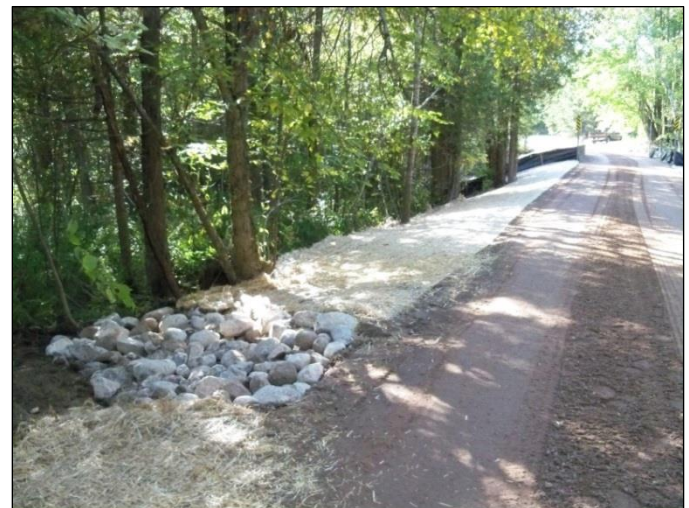
Spillways installed
