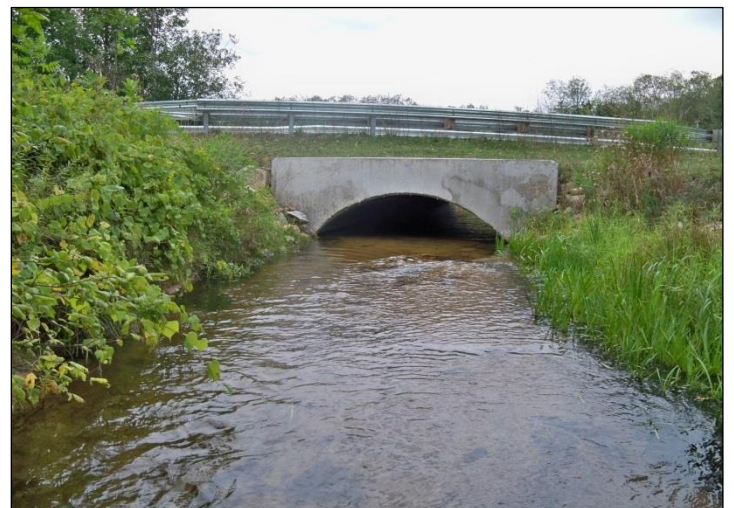
Before – Perched triple culverts upstream of dam. After – Bottomless arch allows fish passage
