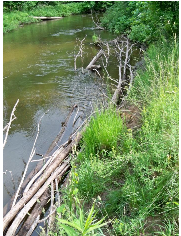
Before & After of embankment erosion along Old King Road. Woody debris, cover structures and rock protect the bank and provide instream habitat for fish and wildlife.
