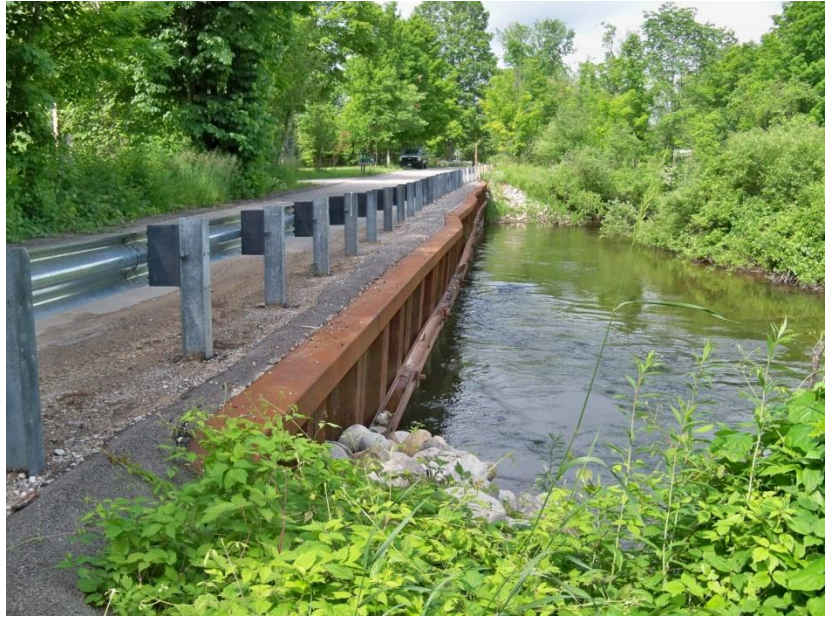
Before & After –Old King Road runs along the Betsie mainstem & served as an access to the former sawmill on Dair Creek. The road was continuously washing into the stream. Sheet piling, fieldstone and pavement now control runoff and stabilize the sensitive embankment.
