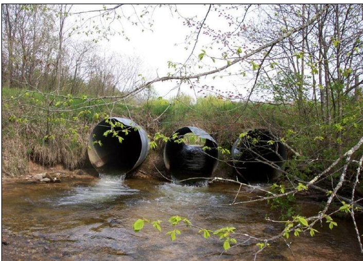
Before – Perched triple culverts upstream of dam. After – Bottomless arch allows fish passage
