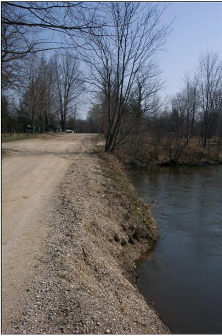
Before & After –Old King Road runs along the Betsie mainstem & served as an access to the former sawmill on Dair Creek. The road was continuously washing into the stream. Sheet piling, fieldstone and pavement now control runoff and stabilize the sensitive embankment.
