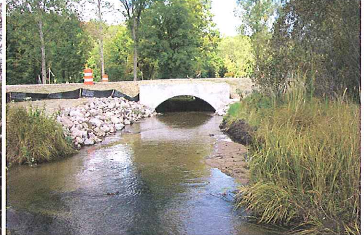
After - Bottomless arch allows fish passage.
