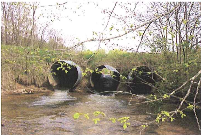
Before - Perched triple culverts upstream of dam.
