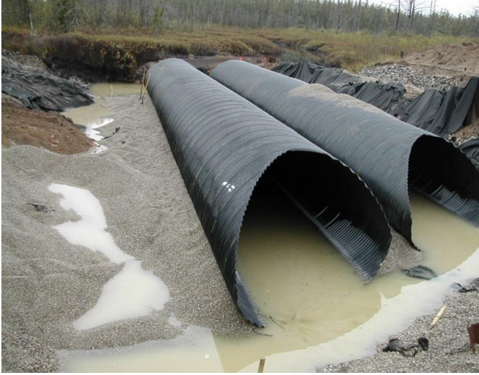
New dual culverts with poly coating placed in alignment with river and finished construction November 2007
