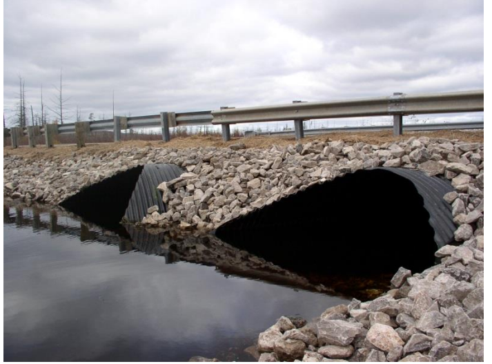
New dual culverts with poly coating placed in alignment with river and finished construction November 2007
