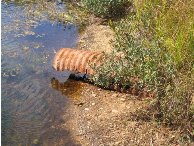
Failing culverts prior
