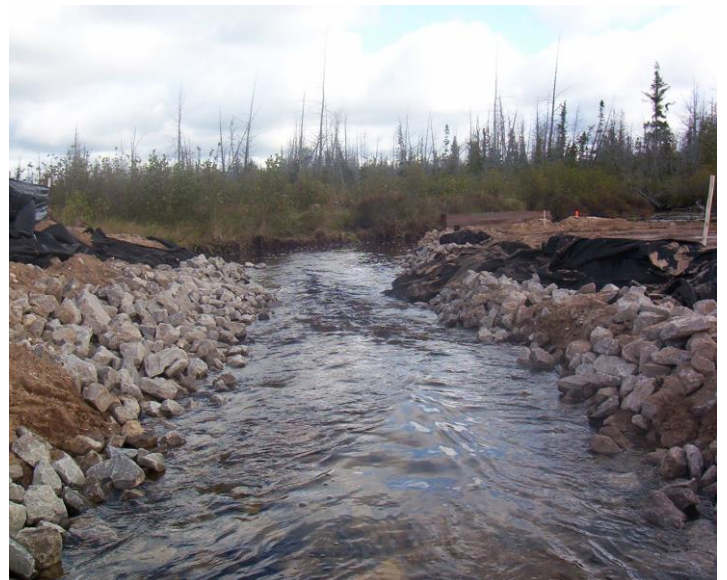
Temporary stream diversion for culvert removal and replacement during construction
