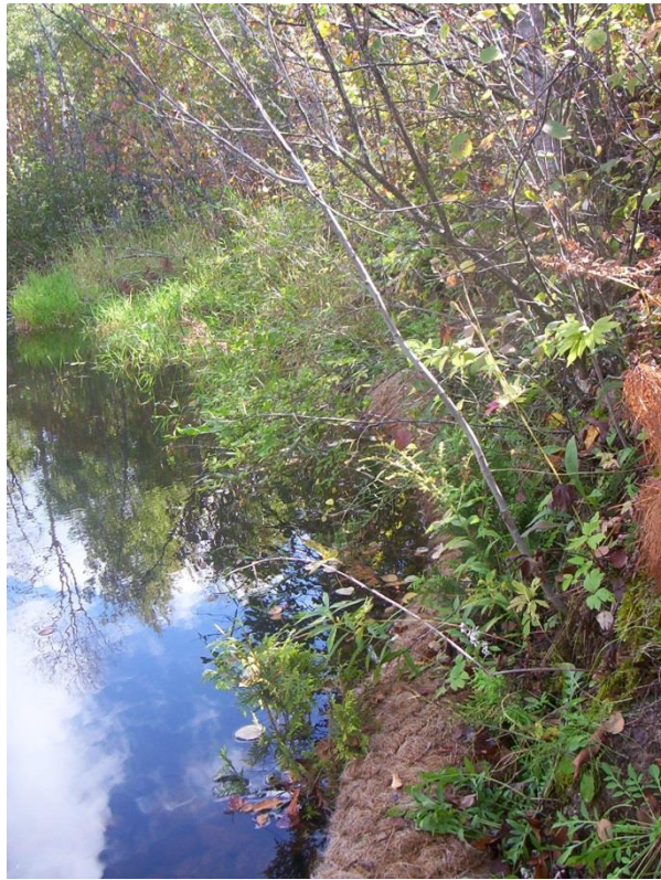
Biologs, fieldstone rip rap, and tree revetments used to stabilize the stream bank
