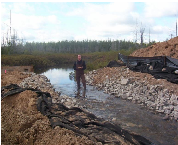
Temporary stream diversion for culvert removal and replacement during construction
