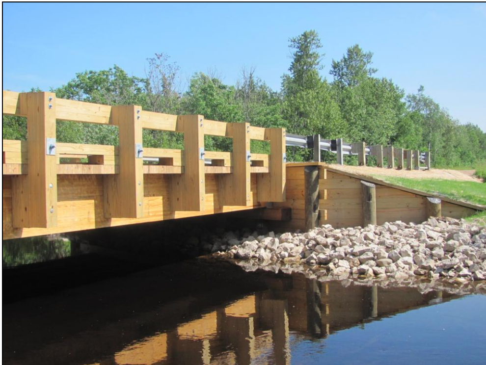
New 40' timber bridge structure allowing aquatic species passage and unrestricted flow.
