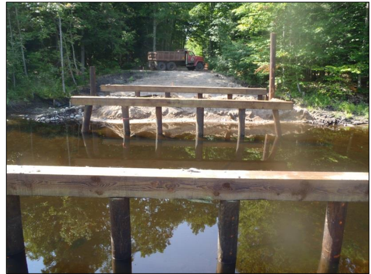
During - Timber piles and abutments were installed
