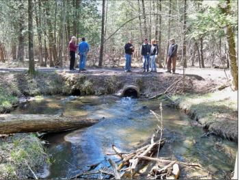
"After" – bottomless arch 10" 11" span, 27' long, 4' 3" rise installed
