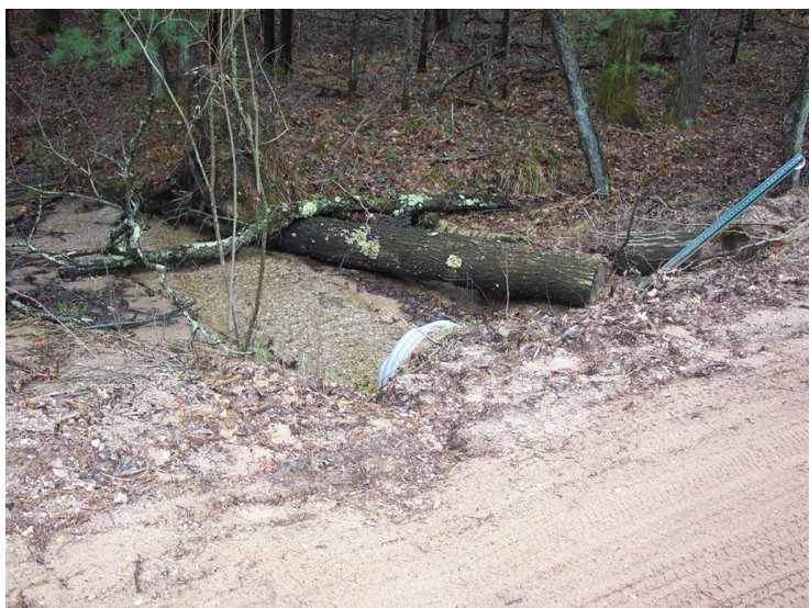
Outlet looking downstream – before
