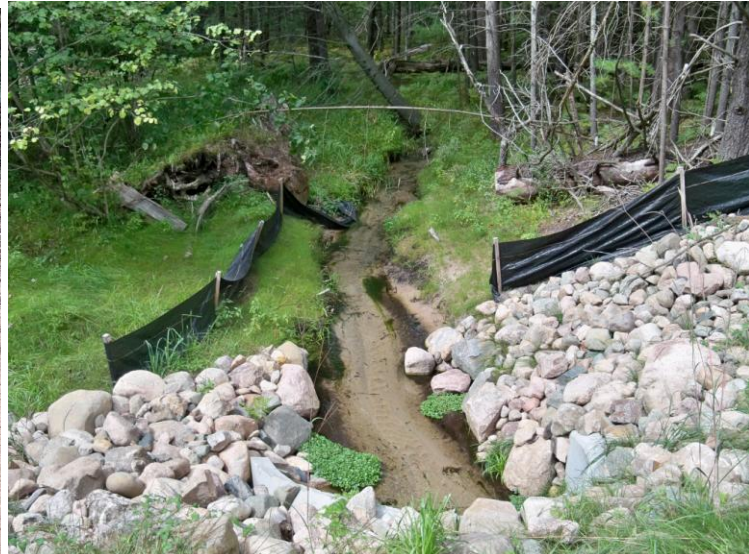
Inlet looking upstream - after
