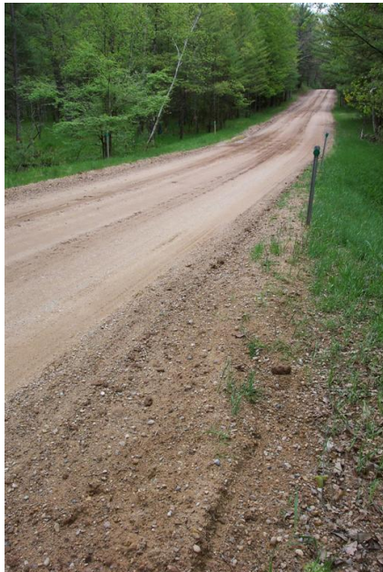
Eroding shoulders – Before
