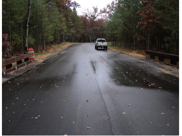
Paved approaches, curbing – After
