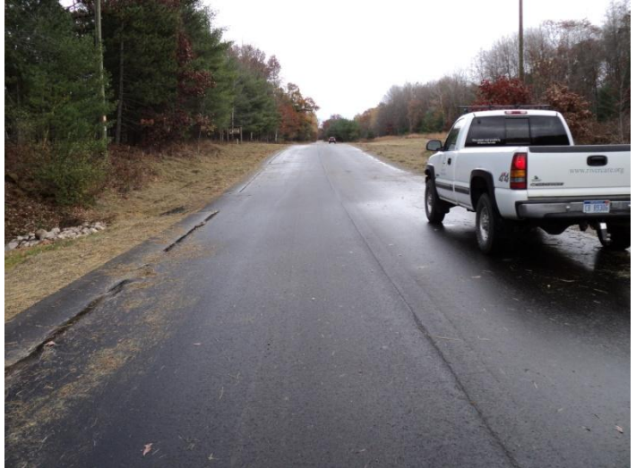
Paving & curbing – After
