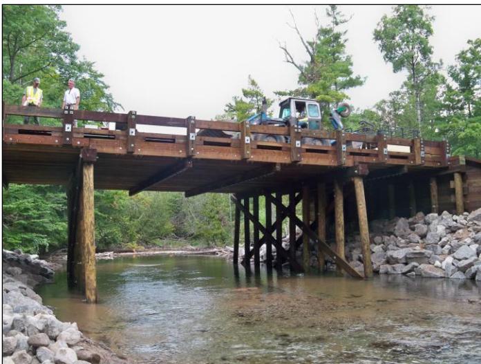
Rock protects abutments from scouring & 1,200' of approach work improves safety & channels road runoff
