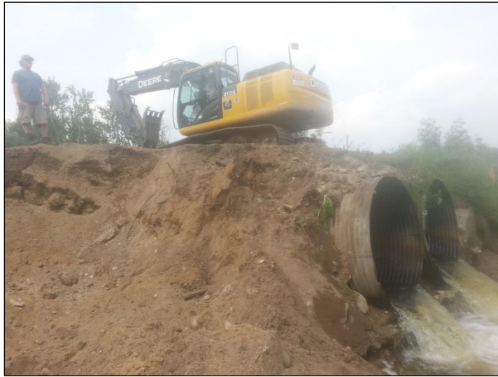
During - The culverts and old roadbed were removed
