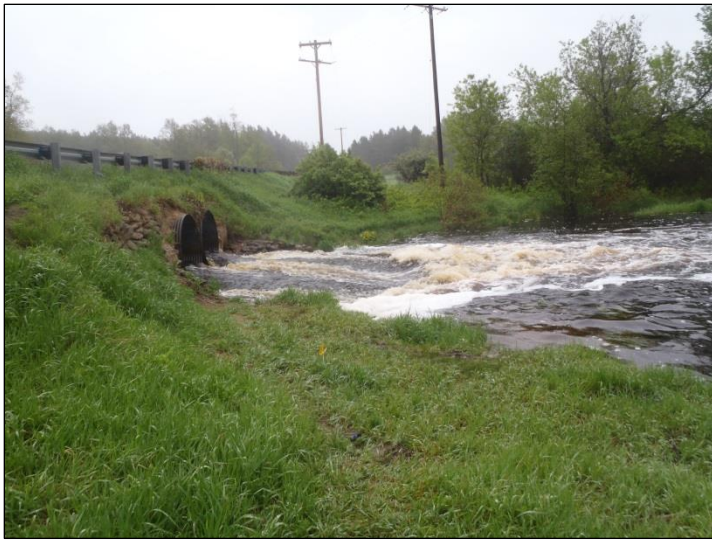
Before - The inadequate twin culverts impeded fish passage and roadbed runoff contributed excessive sediment to the stream
