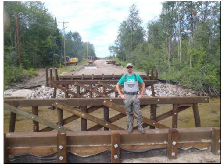
During - Timber piles and abutments were installed
