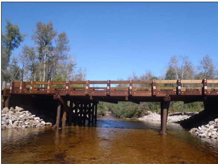
During - The timber deck and restored river channel.
