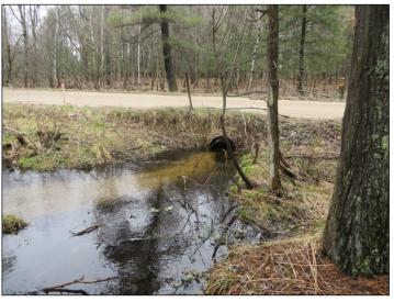
Site #L-67 Before – 2' dia. culvert caused pool formation at the inlet &impounded sediment on this Sanborn tributary
