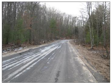
Site #L-67 After – Paved approaches and spillways divert runoff away from the stream & stop erosion of the roadbed
