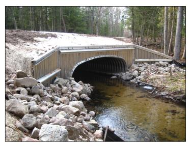
Site #L-65 After – a 16' wide bottomless arch effectively spans Sanborn Creek & allows for a natural stream bottom
