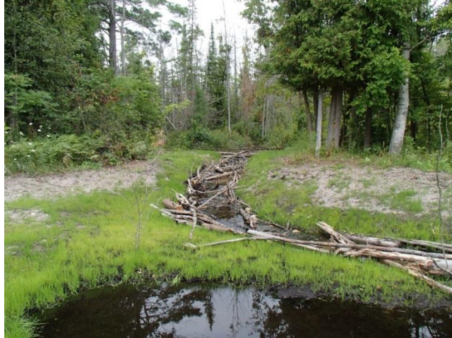
Newly constructed channel
