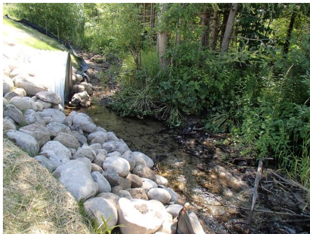
Inlet of new structure at Platte Rd./Brozofsky Creek
