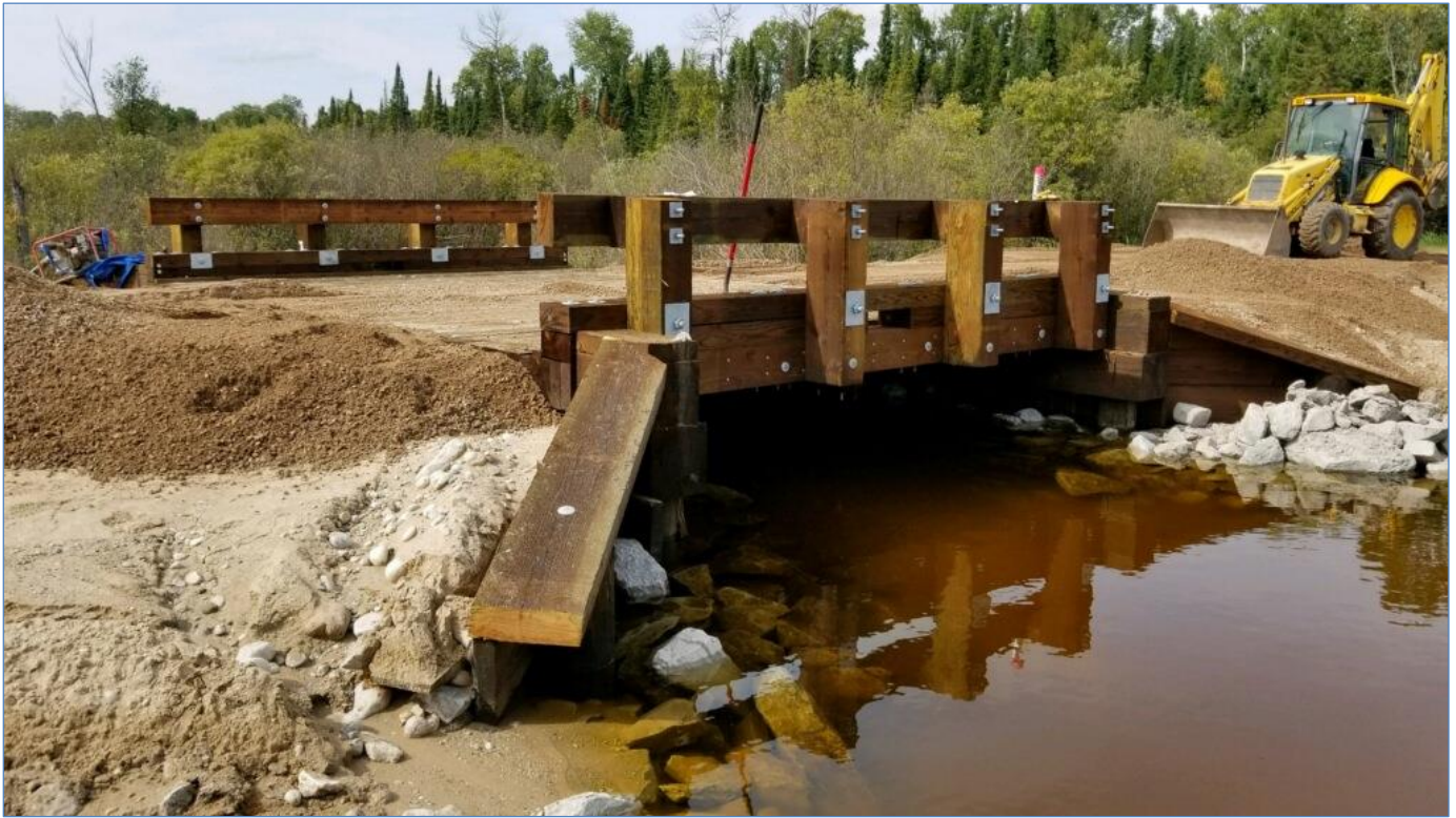
After – Timber deck installed and river channel open for AOP.
