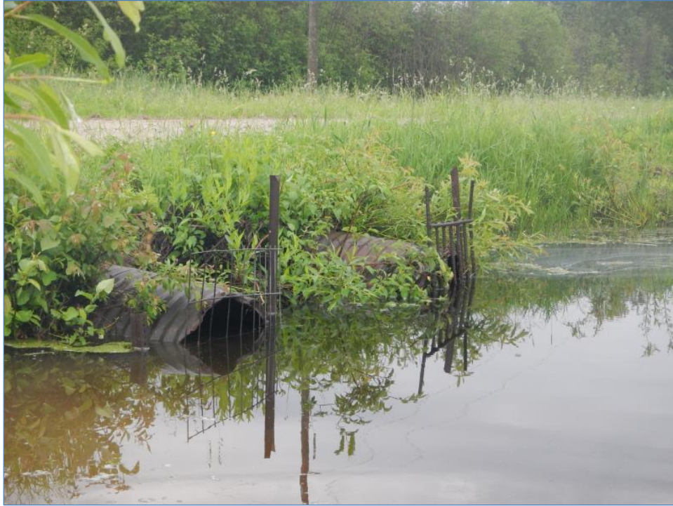
BEFORE – vastly undersized culverts with eroded road embankments
