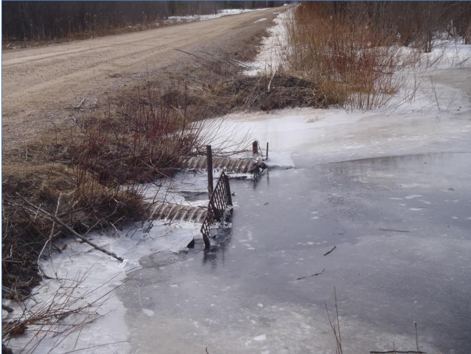
BEFORE – vastly undersized culverts with eroded road embankments
